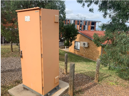
FIG 5 – EXISTING RING ROAD DB SERVICING BUILDINGS ON NORTH SIDE
